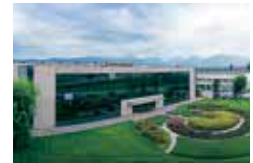
The New Factory
